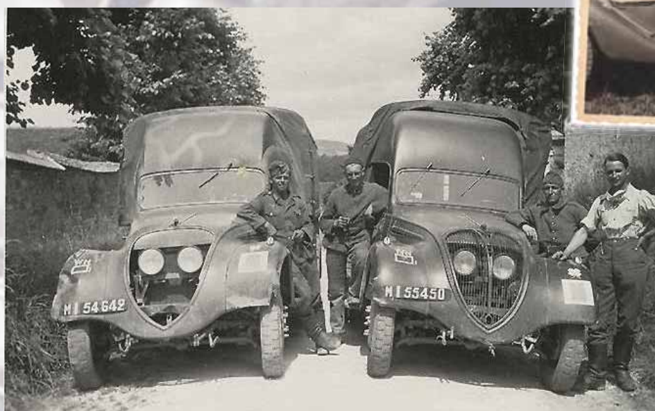
These 402s seem to have larger Michelin tyres and an increased ground clearance.
